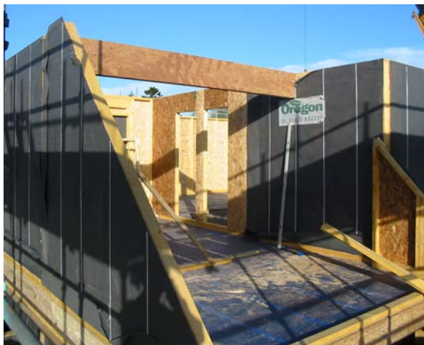
Figure 1: Timber platform frame during construction
