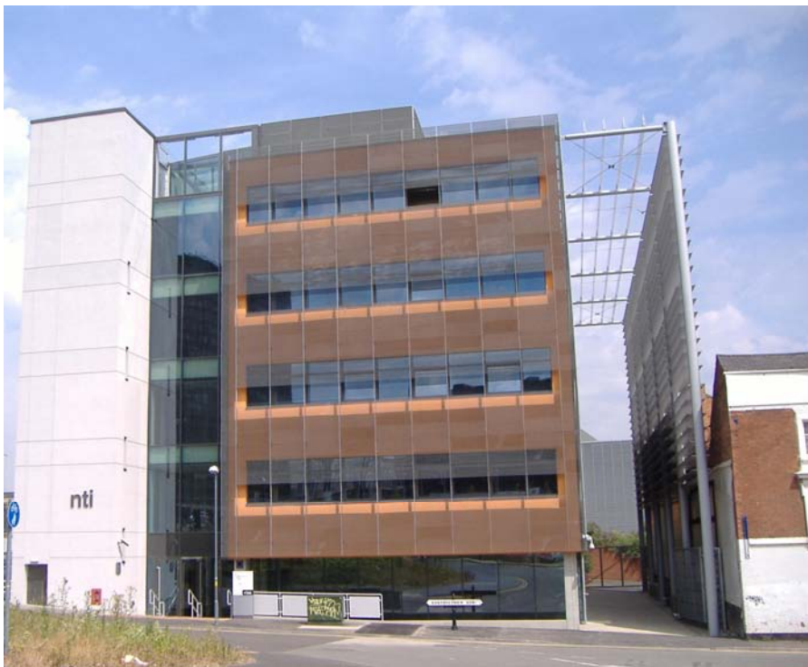
Figure 4 Achieving High Office Standards at the nti Building in Eastside. Metal grills and brille soleil may be seen in front and to right of the building.
